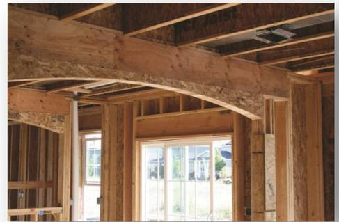
15. The formula to calculate the radius (R) of an arch window is  $R = \frac{W^2 + 4H^2}{8H}$ .
